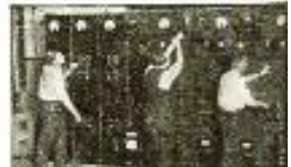
Students at COYNE operating a switchboard that controls power and light enough for a small town
